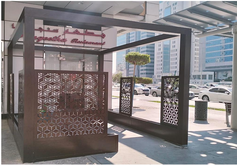
Project: Sangeetha Restaurant, Slam Street Main Contractor: Team Leader General Contracting Description: Aluminum Pergola
