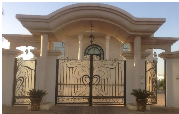
Steel Main Gate
