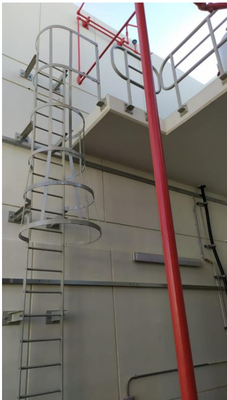
Aluminium Cat Ladder, Handrail & Access Ladder Project: ADDC - AL FOAH - AL AIN
