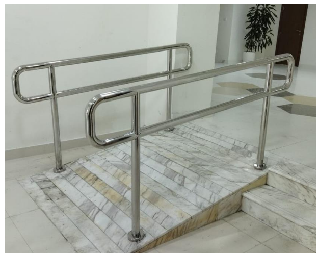
SS Handrail @ Ramp
