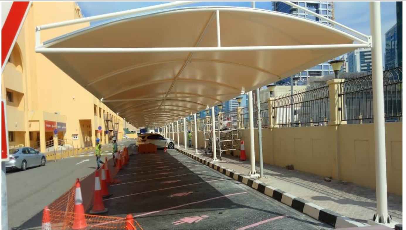
Project: Corniche Hospital , Abu Dhabi Main Contractor: EL Race Construction & Gen. Cont. Co. Description: Car Parking Shade
