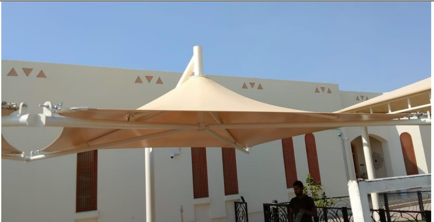
Project: Atfal Al Hilal Kindergarten- Swaihan Main Contractor: Baity Contracting Company Description: Car Parking Shade
